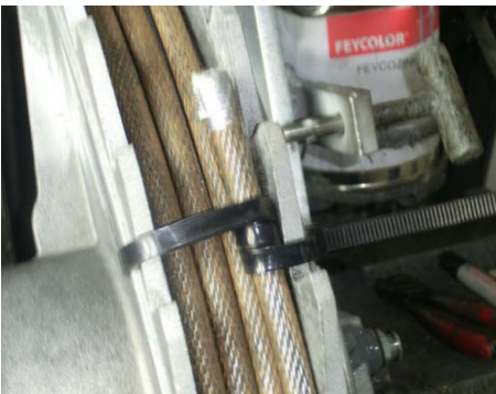
Fig. 21: End of cable secured
