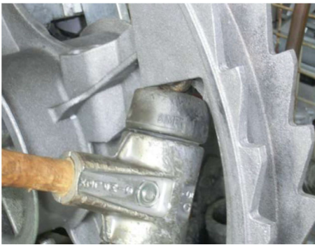
Fig. 20: Hammering in the wedge
